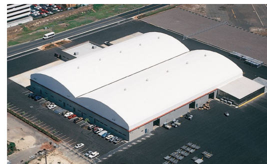
United Airlines uses Shelter-Rite 8028 translucent PVC fabric for 70,000 sq. ft. architectural structure in Honolulu, Hawaii.
