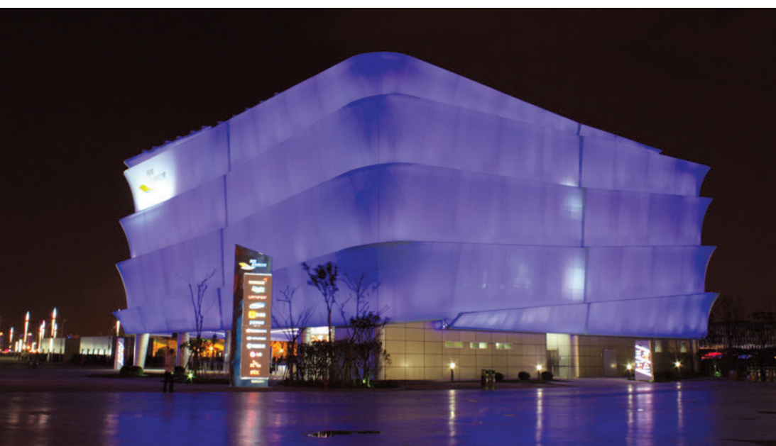
The Shanghai EXPO Korean Enterprise Pavilion facade uses SG-1800 semi-transparent fabric. By MakMax-Taiyo Kogyo Group
