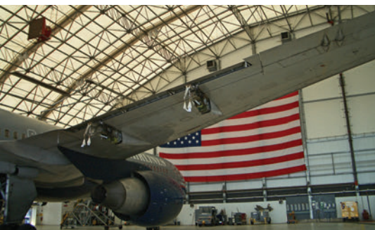
Clearspan structure manufactured by Rubb Building Systems Inc. at Logan Airport uses Shelter-Rite Style 8028 DC-137 translucent PVC fabric with Bright White fluoropolymer coating.
