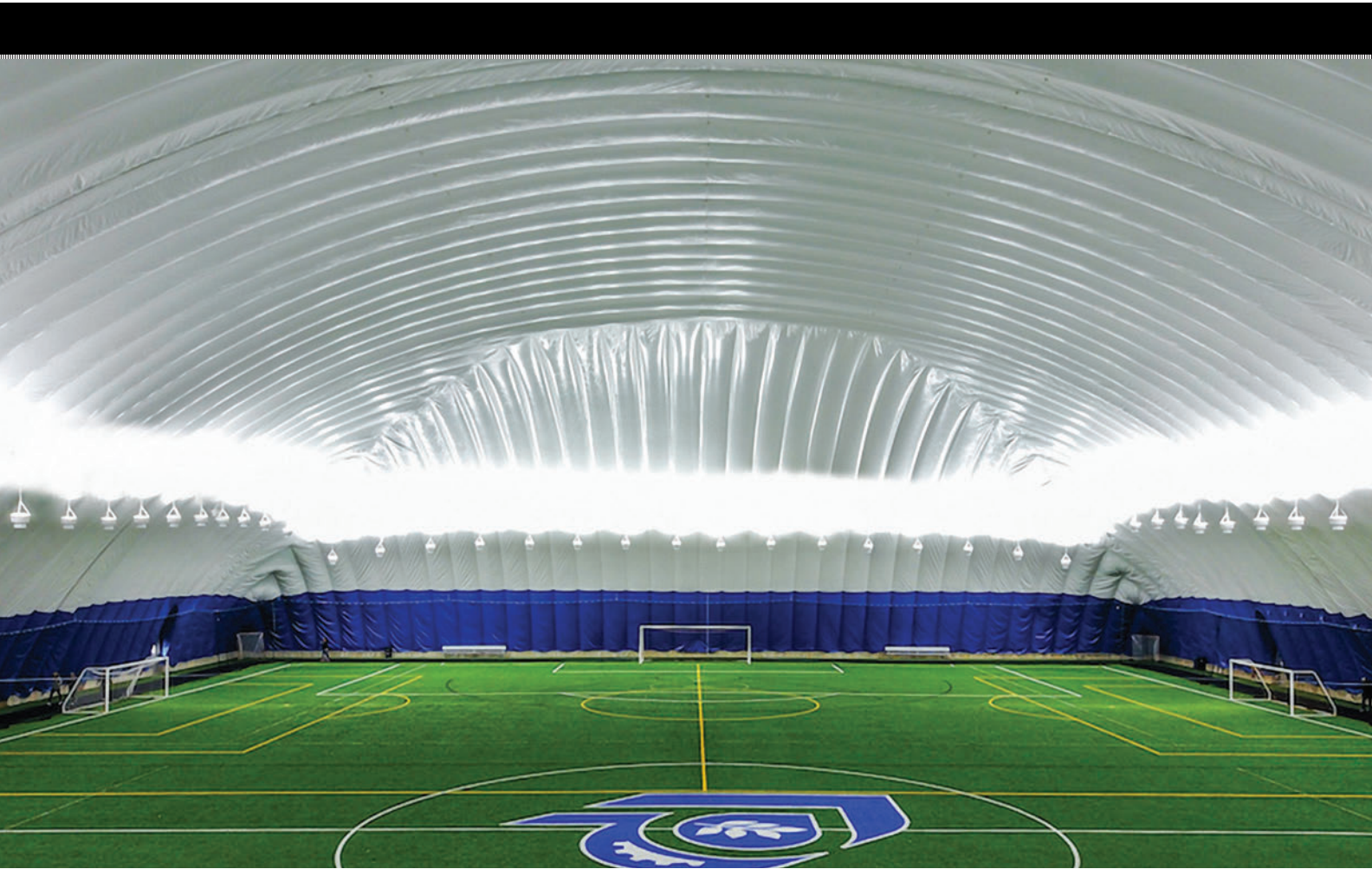
Yeadon Domes used 8028 FRLTC DC4/0/DC6 TS139 71" (PVDF) for this multi-sport dome for Plymouth Parks and recreation in Plymouth, Minn.
