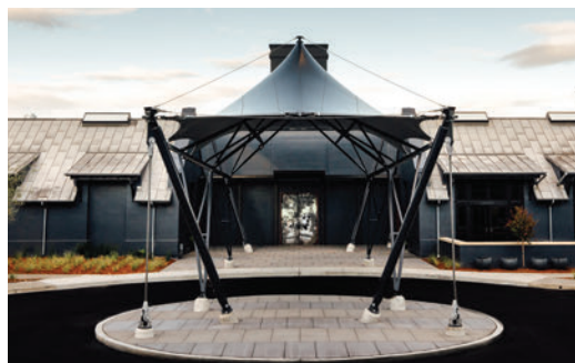
The Prisoner Wine Company, located in St. Helena, Calif., uses 8028 FRLTC, Black/Gray Tedlar for this custom structure by Eide Industries.
