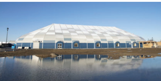
The dual-purpose facility by Sprung Structures for the city of Martensville, Saskatchewan, Canada, and the Saskatchewan Board of Education (Prairie School District) utilizes 9319 FRLTC Colored Tedlar.
