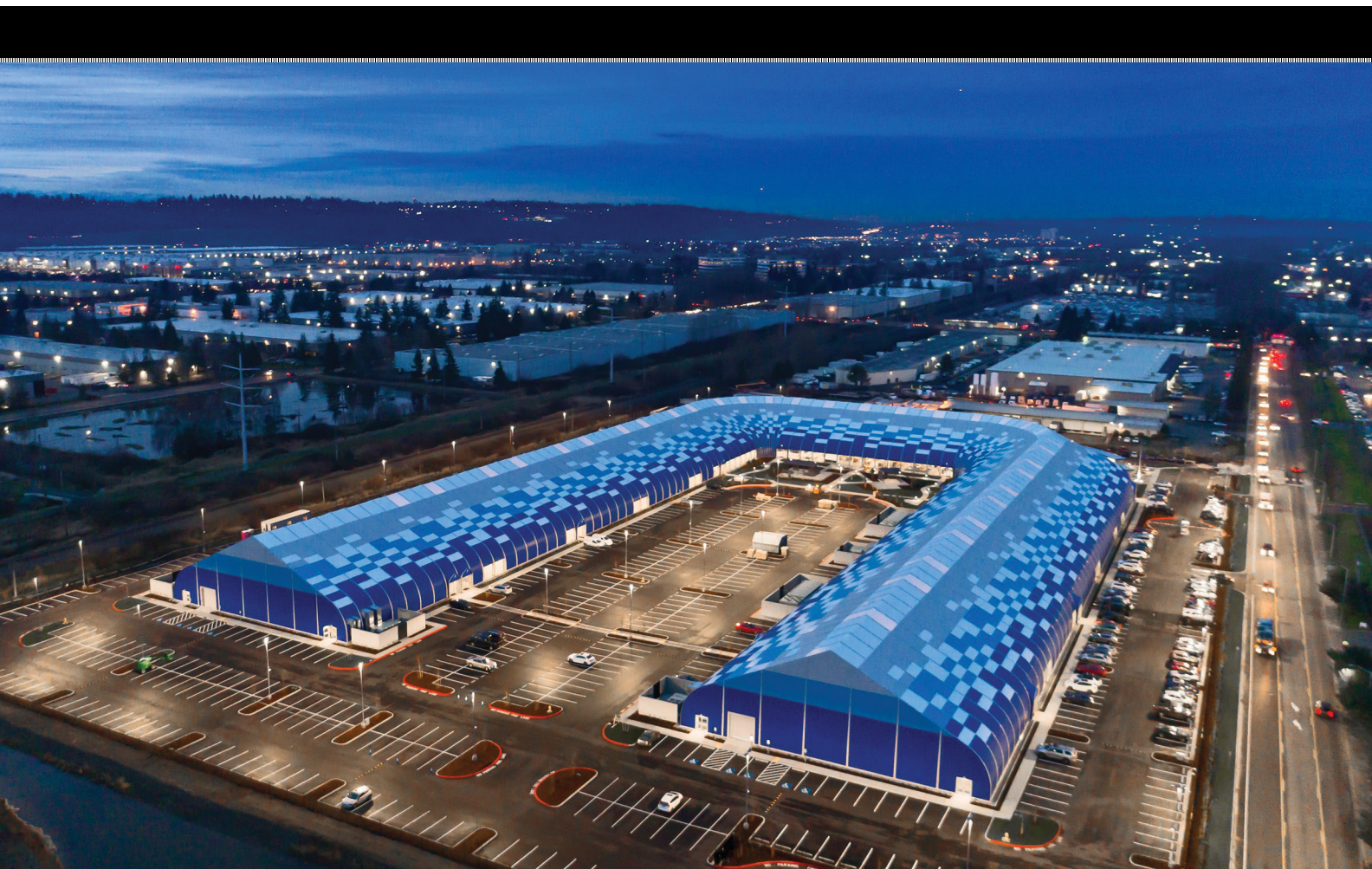
Sprung Structure used Shelter-Rite Style 8324 Kynar and Tedlar Coated Fabrics. Located in Northwest U.S.
