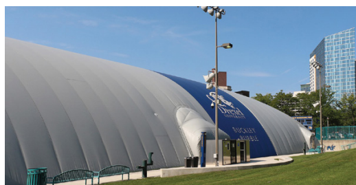
Air-supported structure by The Farley Group uses Shelter-Rite style 8028 with granite gray Tedlar and 8028 blue accent color with acrylic top finish.
